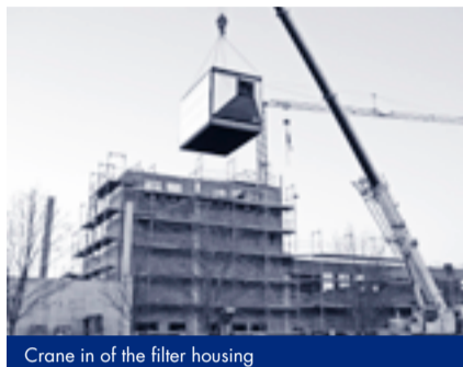
Built-in electrofilter
