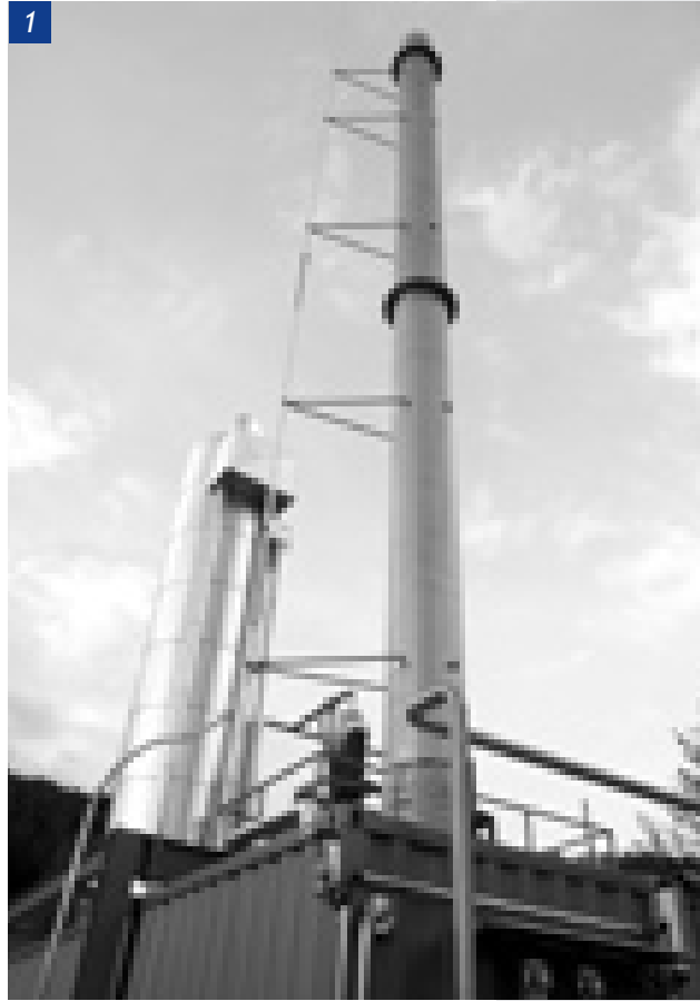
1, 2 Biogas preparation system Leoben
