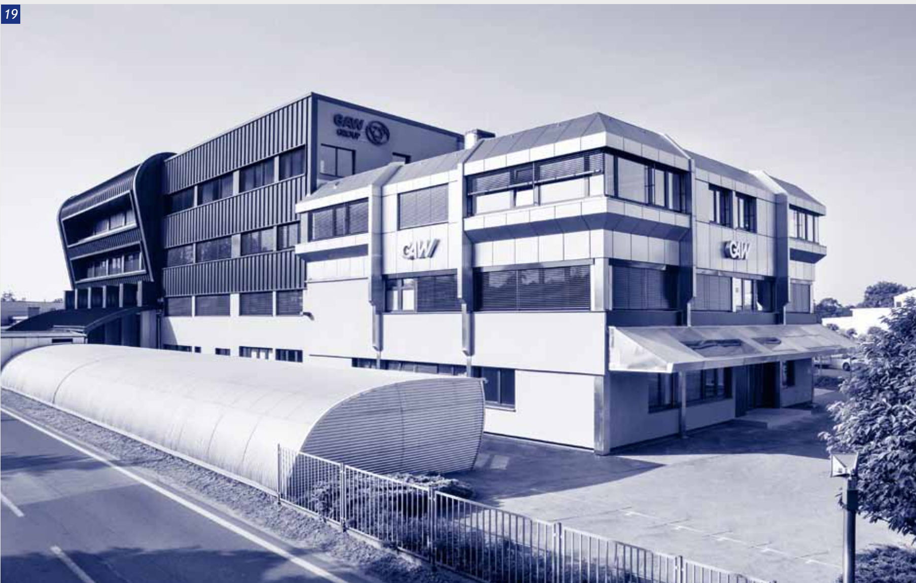
19 The new GAW-headquarter in Graz.
