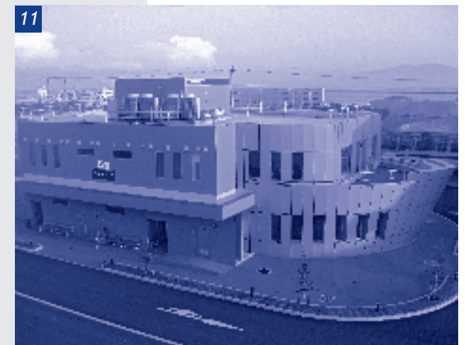
10 Recycling plant CASCADE 11 Start up
