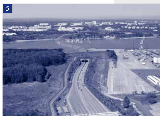
5 The entrance to the almost 800-meter-long stretch under the Warnow
