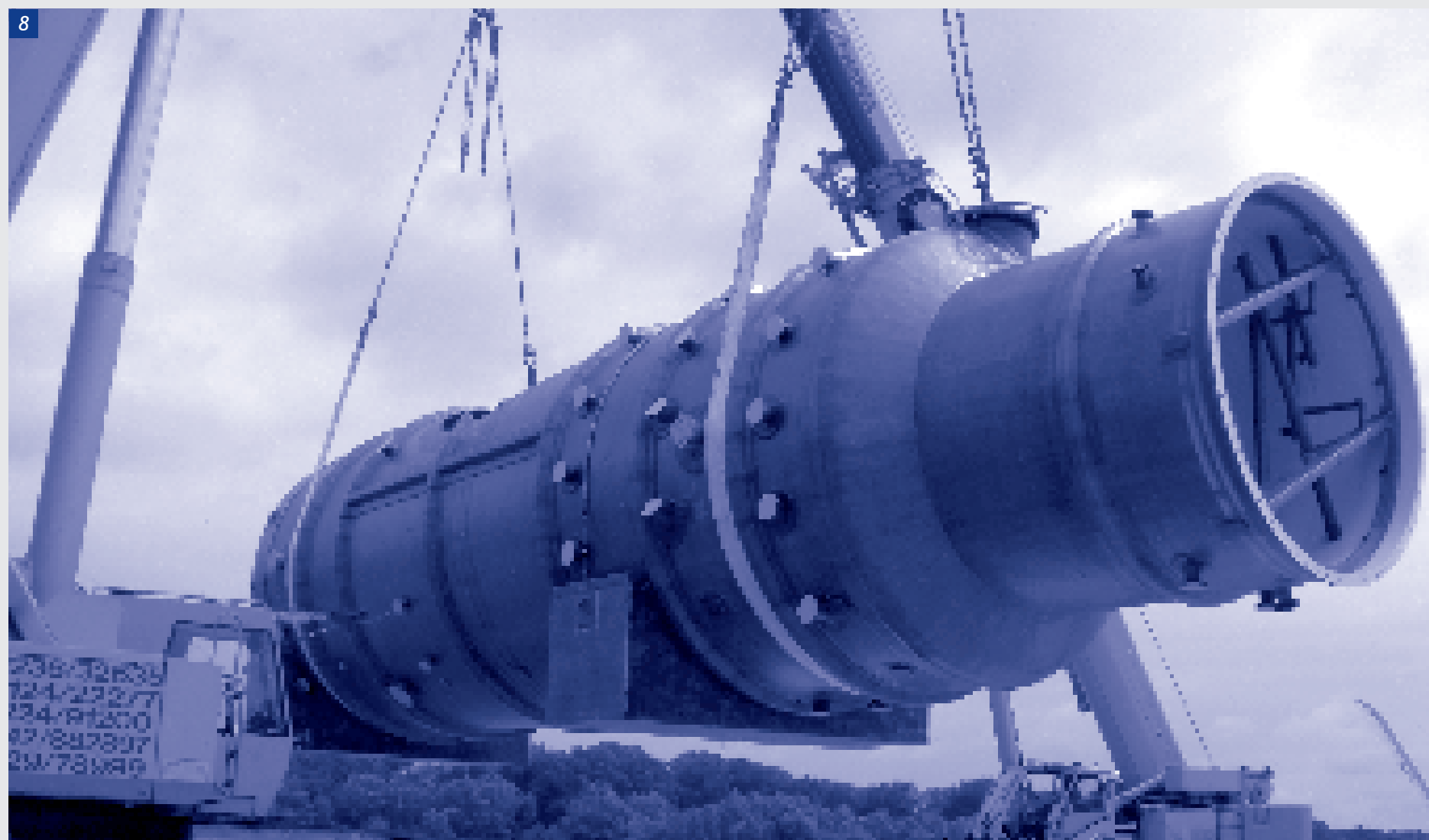
8 Shipment on river ship 9 Special transport via truck to Vienna
